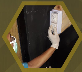
Termite Baiting In-Ground & Above Ground
